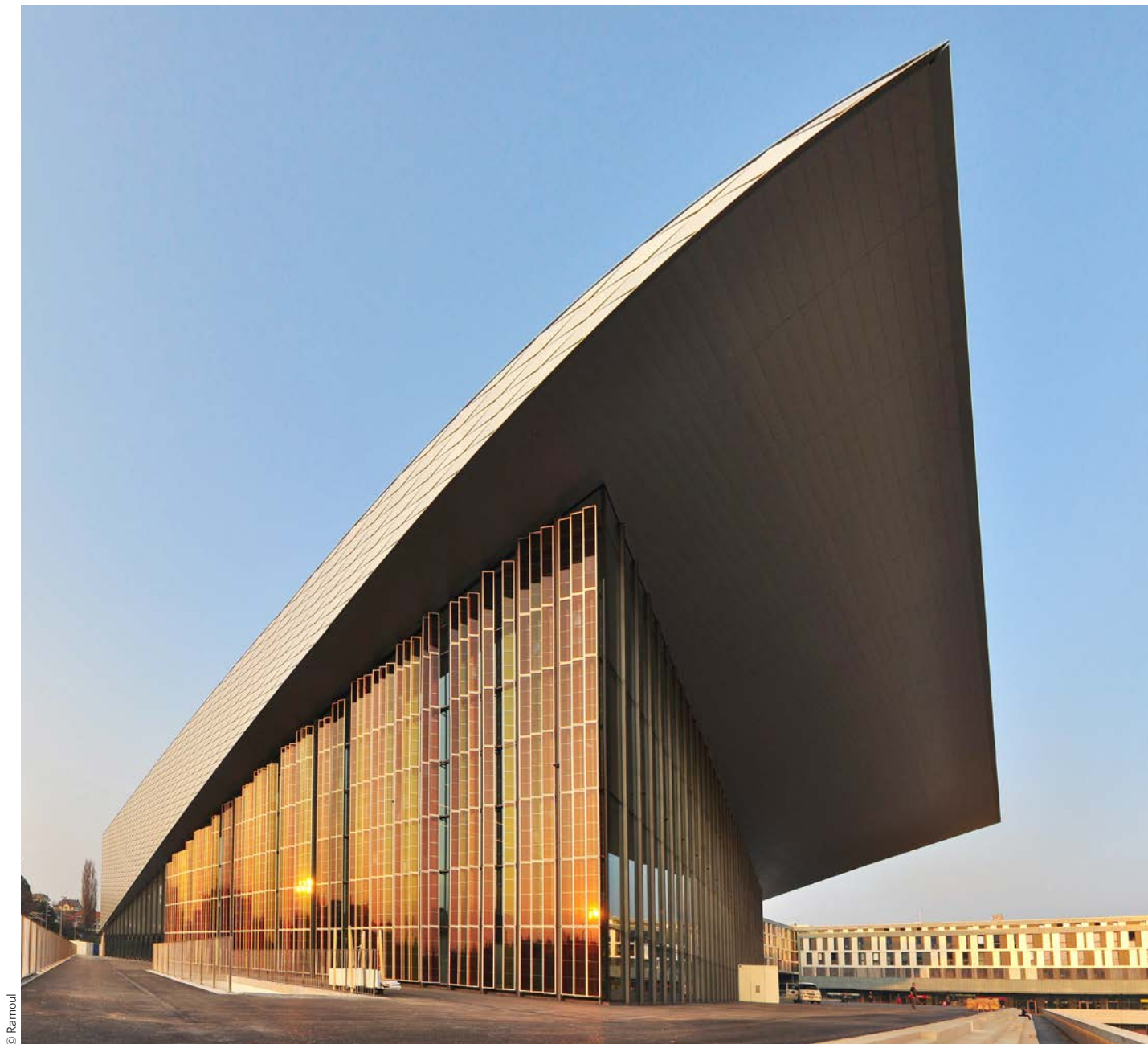
▲ The SwissTech Convention Center in Lausanne, Switzerland. The facade shown is made with panels containing organic dye-sensitised solar cells, a new generation of photovoltaics with great potential
